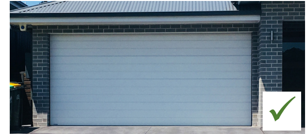
GARAGING - the garage door is not to be a dominant feature of the façade. The garage is to be a maximum of 50% of the width of the façade and is to be set-back a minimum of 1 meter from the main wall of the façade.
