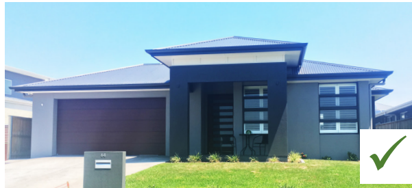
COLOURS - the front façade should incorporate a neutral colour palette with 'tone on tone' colours to add variety.
