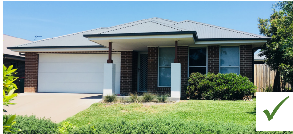
PORTICO - the façade addressing the street is to contain a covered portico which clearly defines the dwelling entry. The portico is to be a minimum of 25% of the width of the façade.
