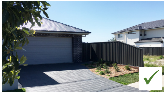
DRIVEWAYS – materials to be exposed aggregate or oxide coloured concrete in dark /neutral tones. Dark grey or charcoal colour preferred.
