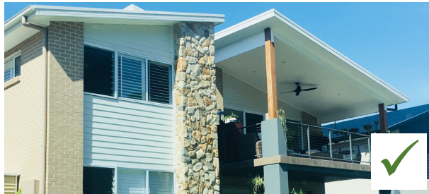
MATERIALS - a variety of building materials are encouraged with a minimum of 2 and a maximum of 3 different materials on the façade addressing the street. Feature stone elements are also encouraged.
