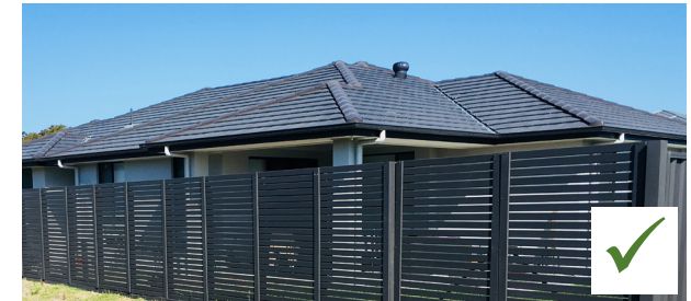
ROOVES - gable or hipped rooves are to be a minimum of 22.5 degrees pitch and skillion rooves a minimum of 10 degrees pitch. Roof materials are to be concrete tiles (flat profile preferred) or metal Colorbond Custom Orb. Roof colour is to be of a natural earth tone with a preference for dark 'grey' tones.
