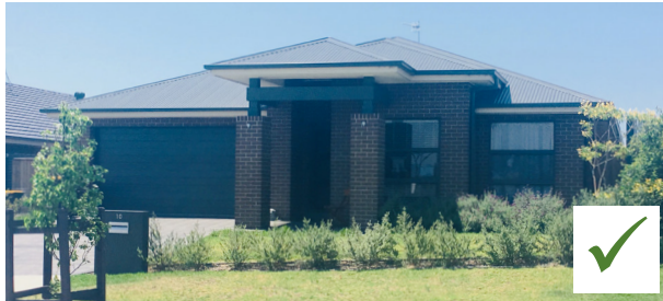
ARTICULATION - the façade addressing the street is to provide visual relief by breaking down the façade into smaller sections. No single wall is to exceed 9 metres in length.
